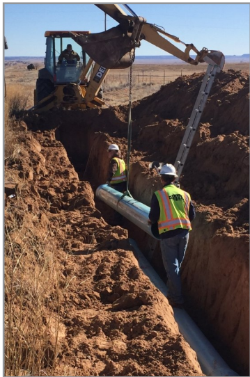
Laying pipe for Freedom II line
