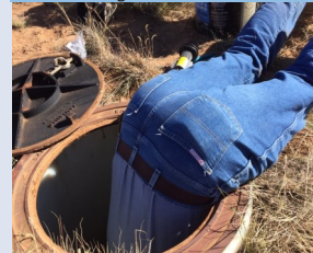
Worn Copper on PRV
