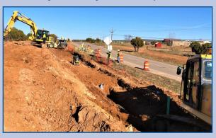
Contractors are finally making progress on the new 16-inch waterline along Frost Road. Weather and wet soil have slowed construction. Any roadways and drainage that are disturbed during construction will be repaired before Entranosa signs off on the project.
