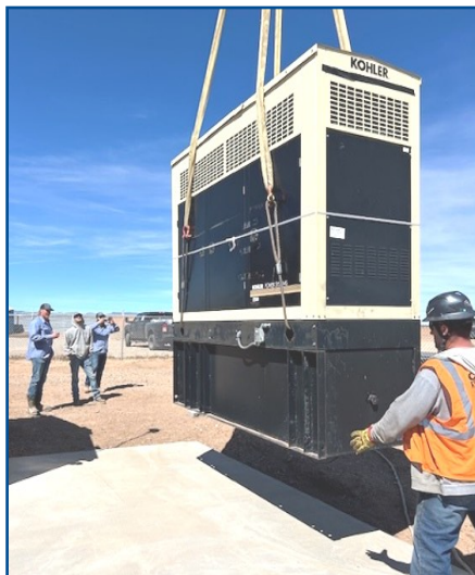
Crane lowers the new generator into place
