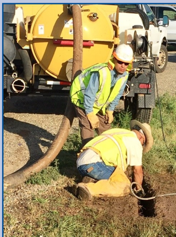
Marking the existing line to install new 16-inch water line
