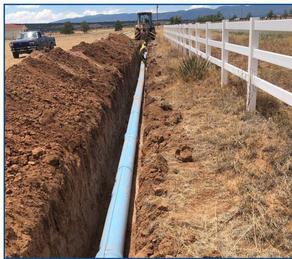
The new 12-inch pipeline along Frost Road
