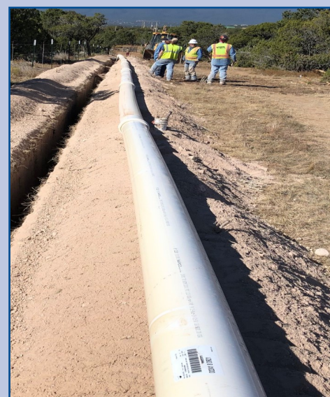
Crews install eight-inch water line
