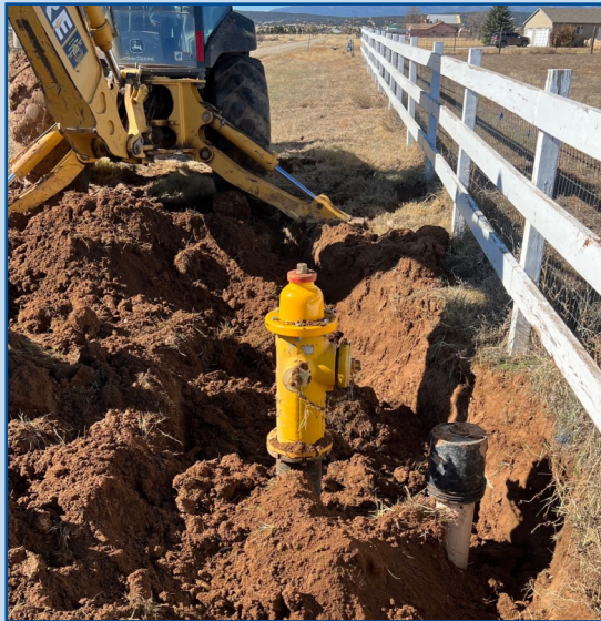
Field Crews Install New Fire Hydrant
