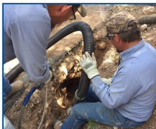
Using the hydro excavator
