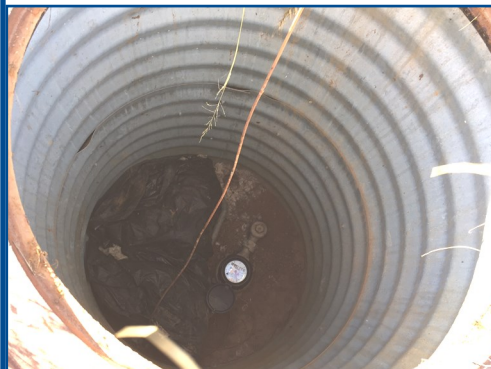
Meter can is 4 to 5-feet deep to protect equipment from frost
