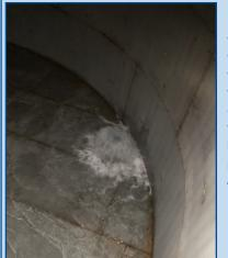
The new Section 6 tank is being filled for a hydro test. In the photo below, the tank is full and overflowing. The tank passed its hydro test and painting begins January 5<sup>th</sup>.
