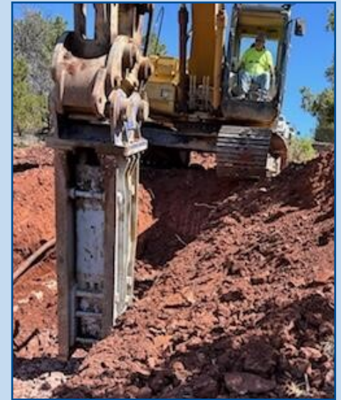
Rock hammer clears the route to the leak
