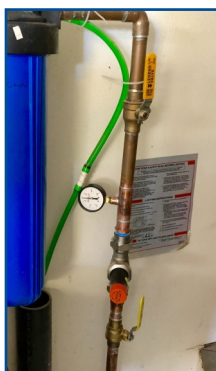
A Pressure Reducing Valve (PRV) helps prevent damage to plumbing from the effects of high water pressure
