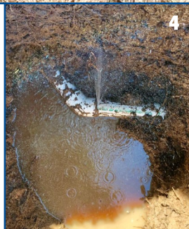
4 — Leak revealed
