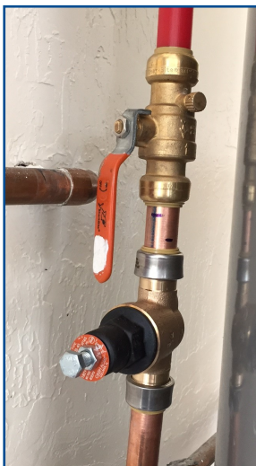
PRV installed in home
