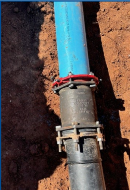
The fix spliced HDPE on to the waterline
