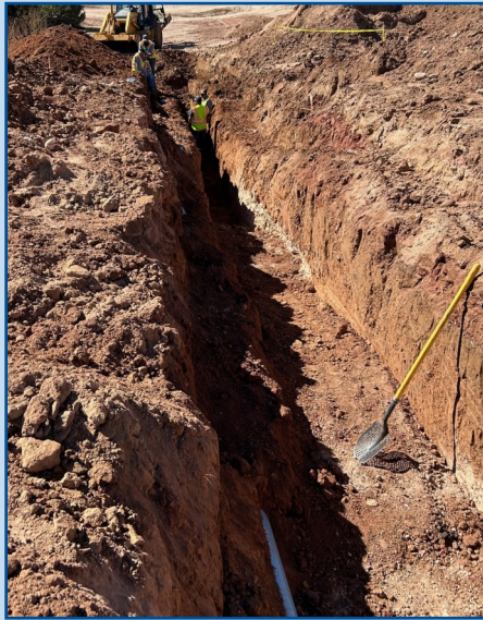
Entranosa's crew digs out 120 feet of waterline
