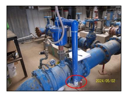
**Recommended Action:** Place a 24-mesh corrosion resistant screen over the air relief blowdown pipe.
